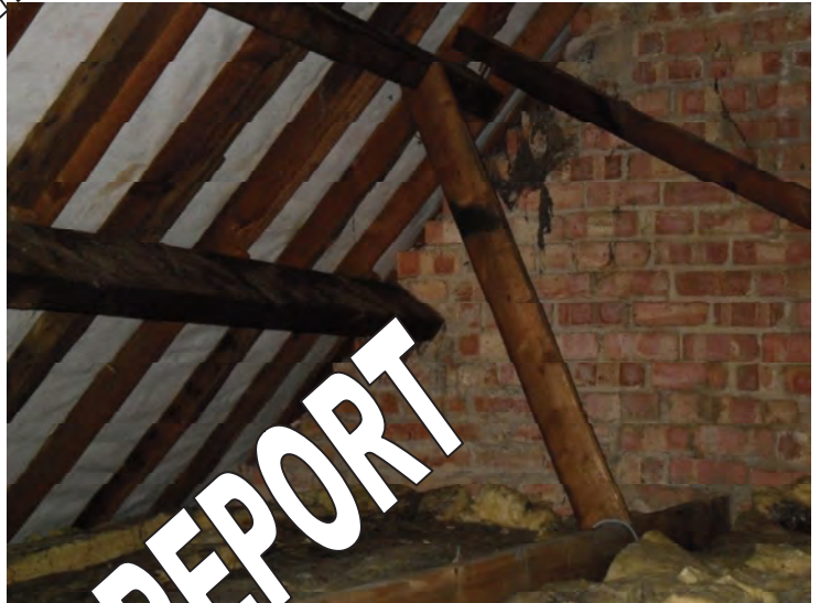
Additional purlin supported by additional struts
